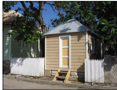
Top: termite damage; before restoration. Middle: Trainee Tony Birthfield on-site; Kenton Nickle working in new shop. Bottom: after restoration.
